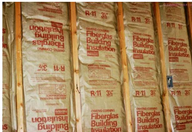
**Photograph 2: Magic Valve** – The asphalt coated kraft facing on the interior side of fiberglass batt cavity insulation changes its vapor transmission according to relative humidity.
