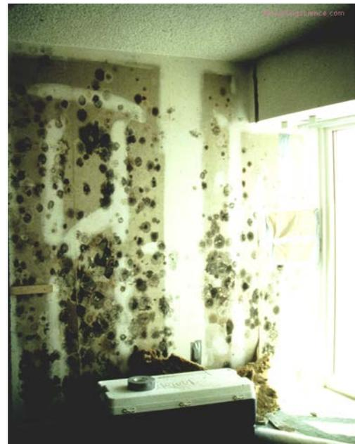
**Photograph 1: Capillary Condensation and Mold** - We can get condensation on porous surfaces at relative humidities less than 100 percent. The condensation occurs in the pores. Mold needs liquid phase water to do its thing yet mold happens on paper faced surfaces at 80 percent relative humidity. Thanks to Lord Kelvin and capillary condensation at 80 percent relative humidity you get liquid phase water in the pores of the paper faced gypsum due to capillary condensation.
