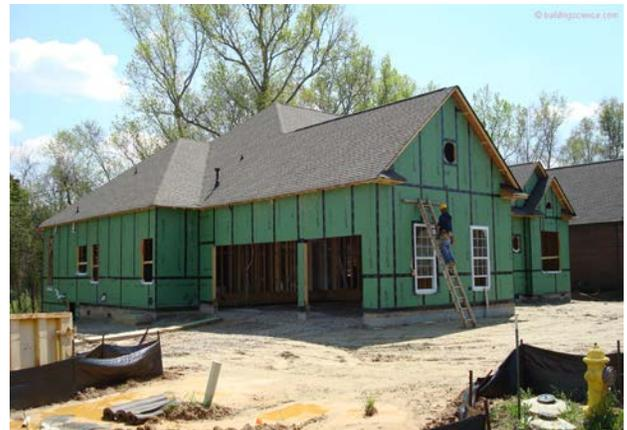
**Photograph 4: Integral Water Resistive Barriers** - It can be argued that the wet cup properties are more significant to performance than the dry cup properties with respect to exterior wall layers.
