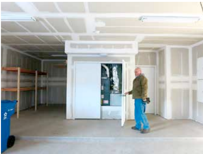
Photograph 5: Sealed Combustion— If the gas furnaces are sealed combustion and the water heaters are sealed combustion then transfer air from the garage is not necessary. Great approach...except... closet gets cold.
