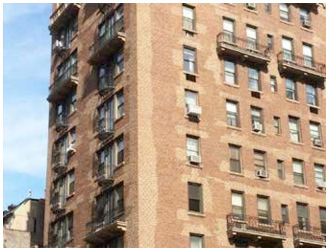
**Photograph 3: Wet Spot Problems**—Where a building gets wet it has problems. Compare this image to **Figure 2**. Guess where all the “repointing” is happening. It gets worse at corners with “pseudo quoin corners”.
