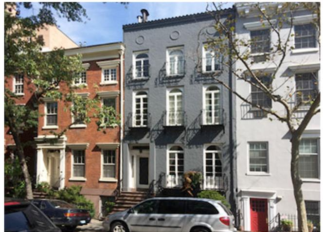
**Photograph 1: “Aging Gracefully”**—Manhattan, Soho, right down town. What’s so interesting about this streetscape? The house on the left is brick masonry. The house in the middle is painted brick masonry. The house on the right is stucco over brick masonry. Better and better water control from left to right. Owners figure things out.
