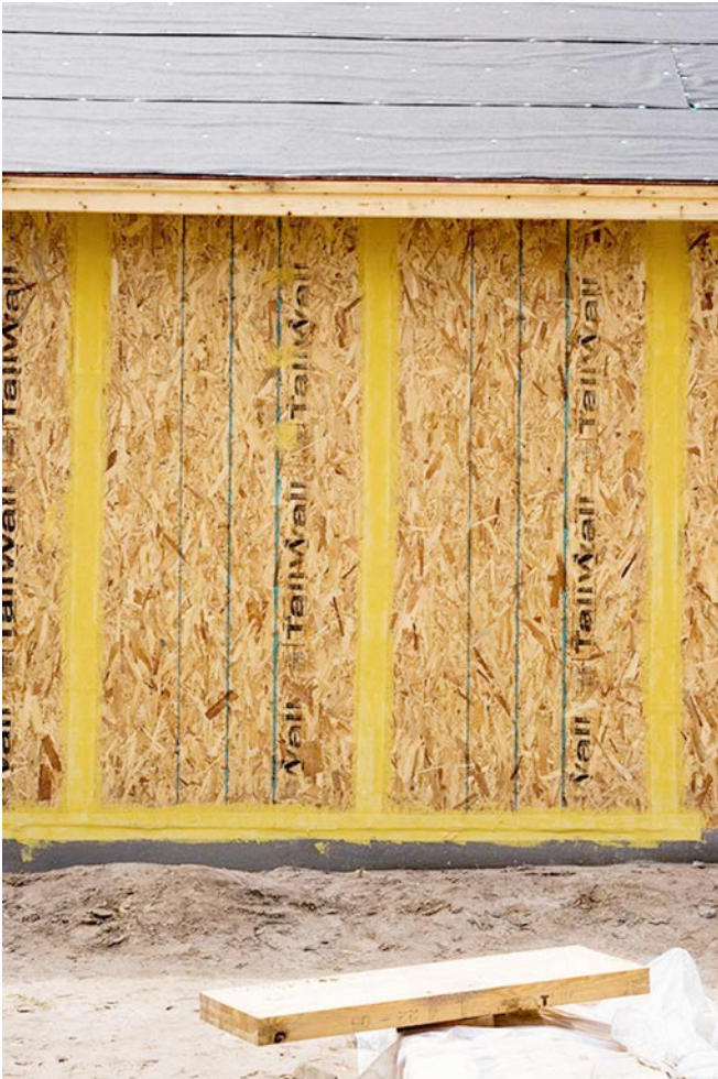
Photograph 15: Fluid Applied Joint System —Replacing tapes with fluid applied joint systems is now possible.
