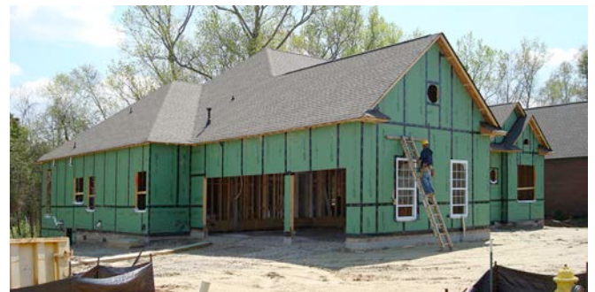
Photograph 13: Sheathing Water and Air Control Layer— The sheathing in this system is pre-coated with a water control layer. Tape is used provide water control and air control layer continuity.
