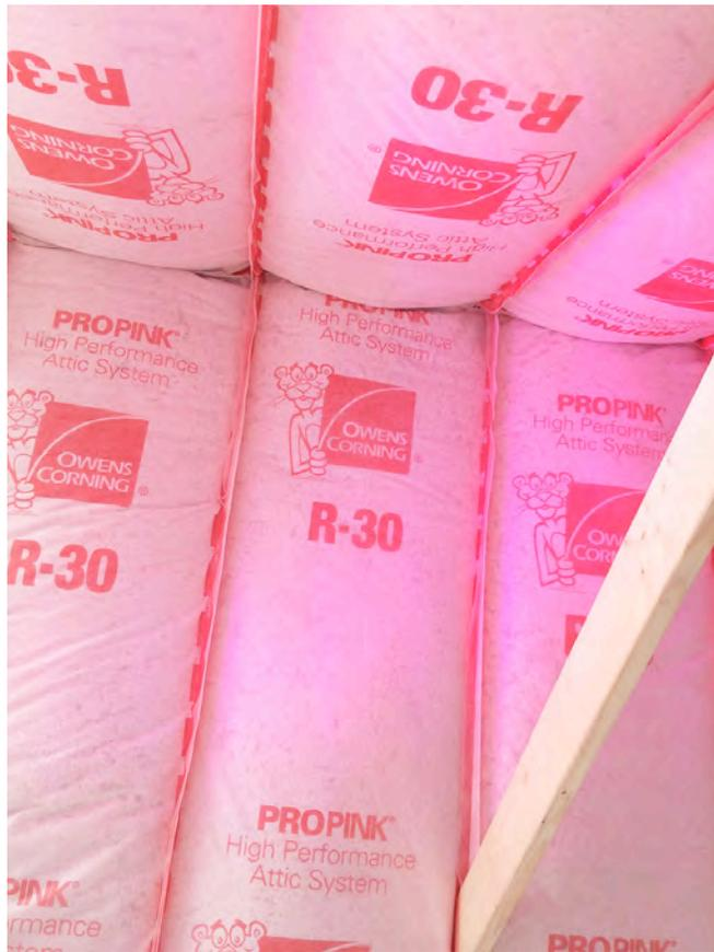
**Photograph 14: Blown Fiberglass—**Works with fiberglass blown into a netted semi permeable sheet.
