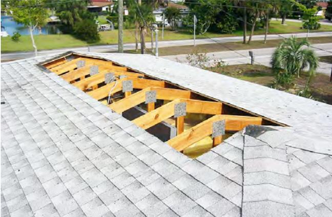
**Photograph 4: Solar Dehumidifier** – How big should the vent be? Just guess. Turned out to be twice as big as necessary. Limiting factor was not the diffusion vent area but getting moisture from the house into the cellulose.
