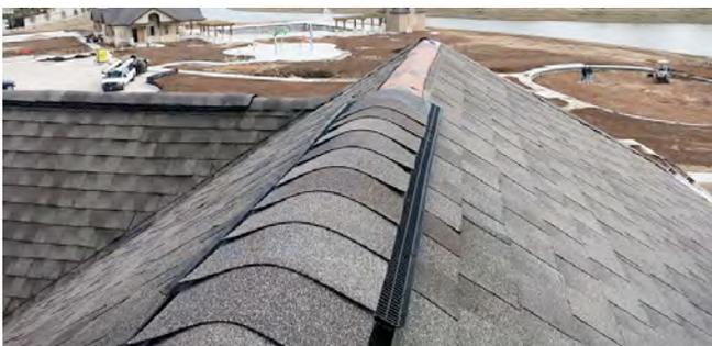
**Photograph 10: Ridge Vent—**Off-the-shelf shingle covered ridge vent works just fine.
