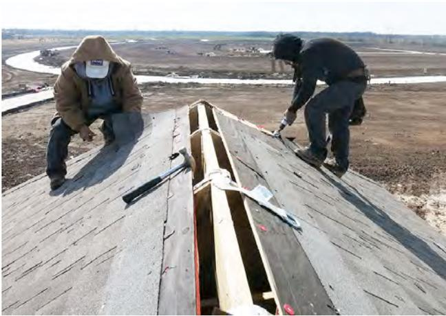
**Photograph 8: Vent Opening In Roof Sheathing—**Standard construction practice is used to provide vent opening at ridge area.
