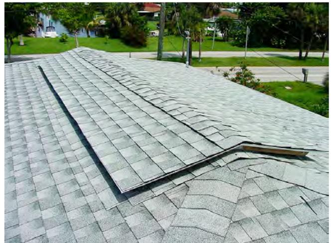
**Photograph 7: End of Solar Dehumidifier** – A glorious attempt. Works well enough to keep the roof from rotting but not well enough to address part load humidity problems in energy efficient houses.
