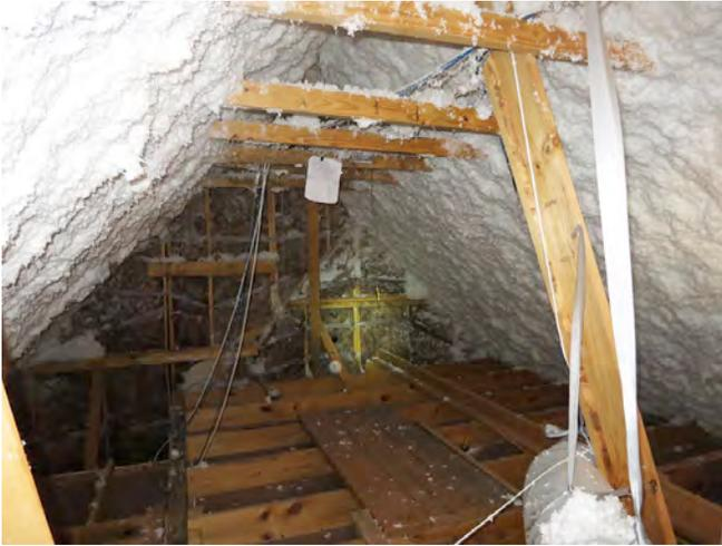
**Photograph 13: Adhesive Spray Applied Fiberglass—**Yup, works here as well.
