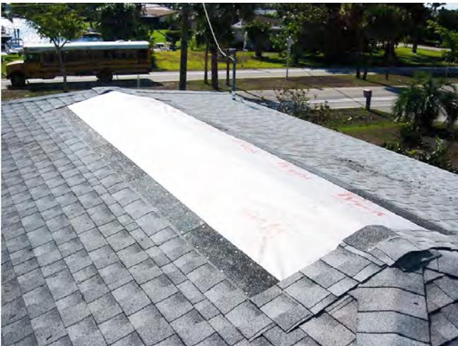
**Photograph 5: More Solar Dehumidifier** – Water tight, air tight but vapor open membrane.
