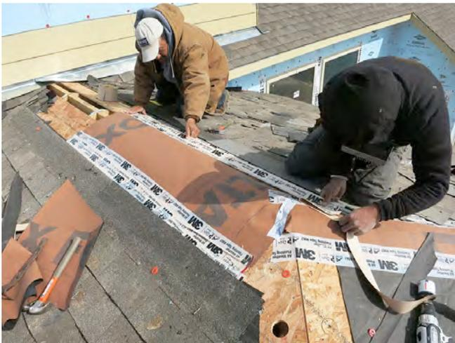
**Photograph 9: Vapor Open Membrane—**Commercially available house wrap/building wrap used to cover vent openings in roof sheathing.
